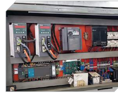
Elektrik panosu Electric panel
