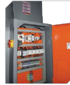
Elektrik panosu Electrical system board
