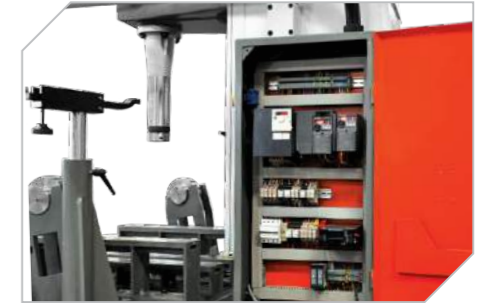
Elektrik panosu Electric panel
