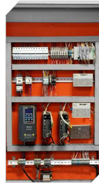
Elektrik panosu Electric panel
