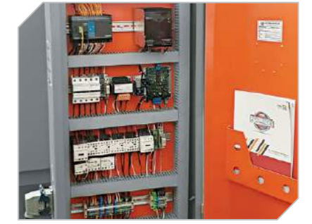
Elektrik panosu Electric panel
